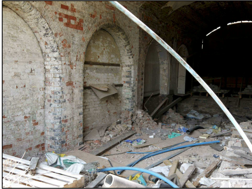
VIEW OF VAULTS CONTAINING CROSS ARCHES Vaults to be opened up and cleared of rubble to enable existing cross arches to be surveyed.
